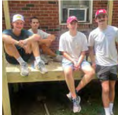
Some FPC youth & young adults helped build a ramp in July.
